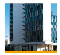
The building contains 361 bed spaces in 36 clusters, including 217 studio flats. With 11 floors of light gauge frame sitting upon a first floor podium, Sigmat believes this is currently the UK's tallest completed light gauge steel frame building. The Sigmat team completed the multi-level scheme in just 17 weeks.
